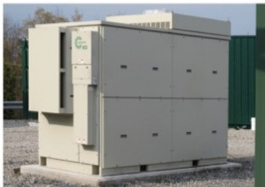
Coal Bed Methane Gas Processing Plant, Charleroi, PA C200 Microturbine in a distributed generation application
