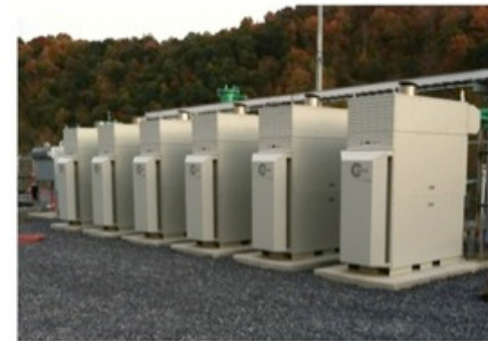
Gas Compression Site, WV Six C65 MicroTurbines provide all onsite electricity & heat for fuel gas conditioning
