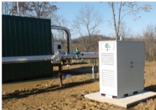
Meter & Relay Site, Proctor, WV C30 MicroTurbine in a wellhead gas application
