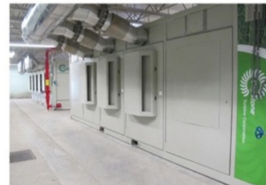
Wastewater Treatment Plant, York, PA Biogas-fueled CR600 in a CHP application & a natural gas-fueled C1000 in a peak shaving dispatch application
