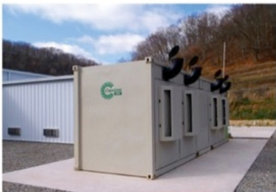
Water Pumping Facility, Cameron, WV C800 Power Package providing provides all onsite electricity
