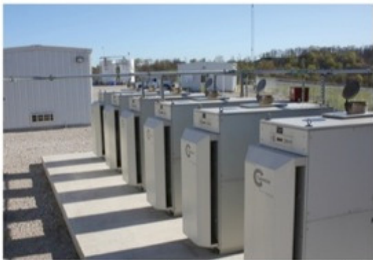
Gas Gathering & Compression Station, Marshall County, WV Six Capstone C65 MicroTurbines generate all onsite electrical power
