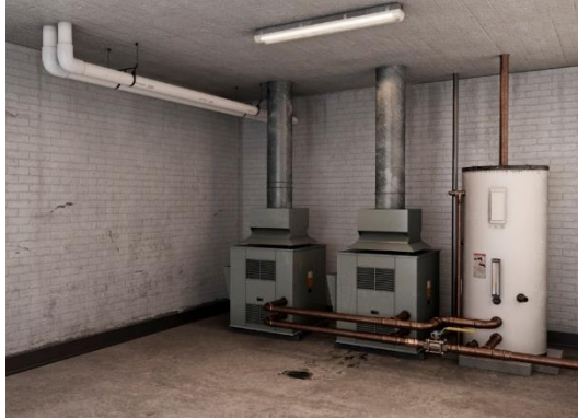
Existing Boiler Room
