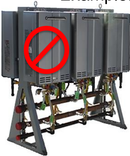
One Rinnai tankless disabled: loss of 16% DHW
